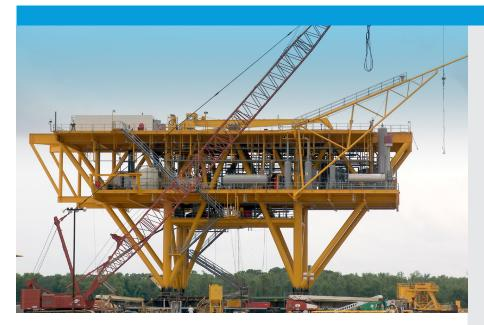
Carbozinc 11 Series are inorganic zinc primers exhibiting outstanding corrosion and undercutting resistance. Their long-term protection has labeled them as "permanent primers" and has outperformed galvanizing.
