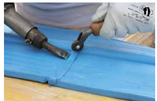
Steps to form a butt weld in Idrostop PVC BI: a) heat the two edges of the bulb with a Leister; b) press the two edges together to form a bond; c) slightly overlap and weld the ends of the rims of the waterstop together; d) final step of the welding procedure; e) apply a strip of PVC to strengthen the welded bulb; f) apply a strip of PVC to strengthen the welded rims of the waterstop
