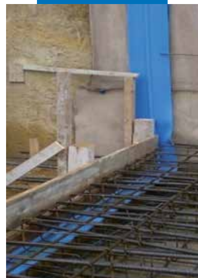
Sealing a structural joint on a vertical wall
