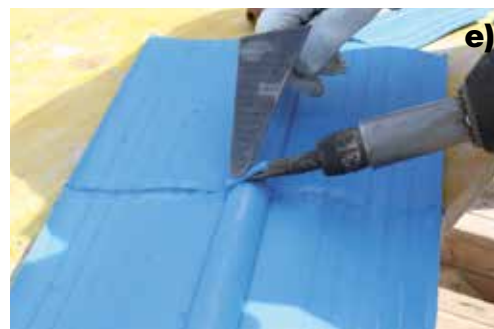
Steps to form a butt weld in Idrostop PVC BI: a) heat the two edges of the bulb with a Leister; b) press the two edges together to form a bond; c) slightly overlap and weld the ends of the rims of the waterstop together; d) final step of the welding procedure; e) apply a strip of PVC to strengthen the welded bulb; f) apply a strip of PVC to strengthen the welded rims of the waterstop
