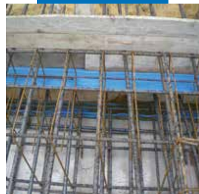
Sealing a structural joint on foundation
