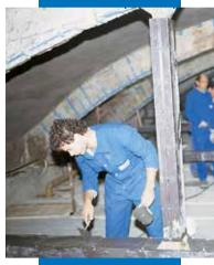
Pouring Mapegrout Hi-Flow into metal formwork
