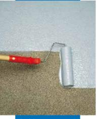
Applying Mapecoat I 24 with roller
