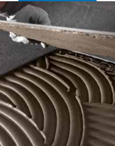
Installing thin porcelain tile on floor
