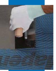
Waterproofing with Mapelastic reinforced with Mapenet 150
